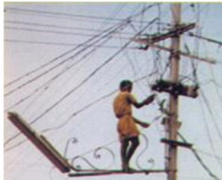
Snapshot of illegal hooking from the network
