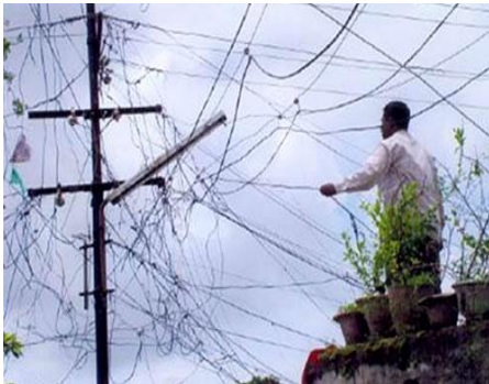
Snapshot of illegal hooking from the network
