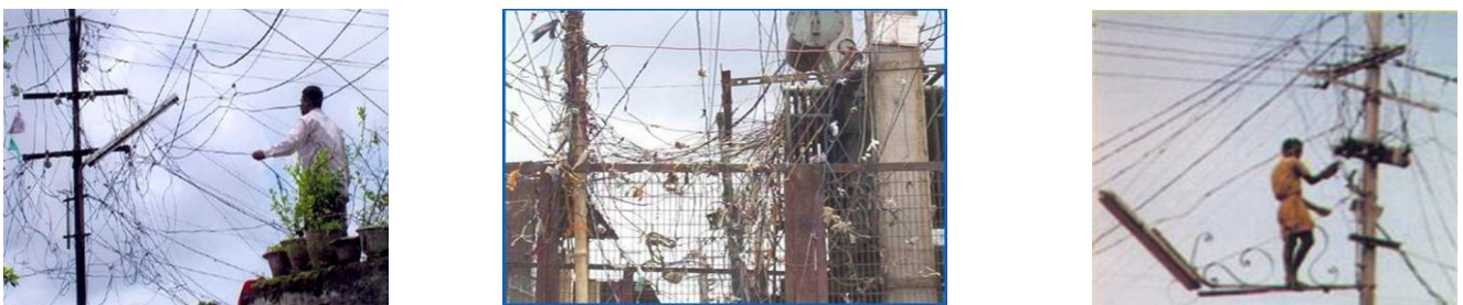
Fig 2: Illegal hooking from the network
